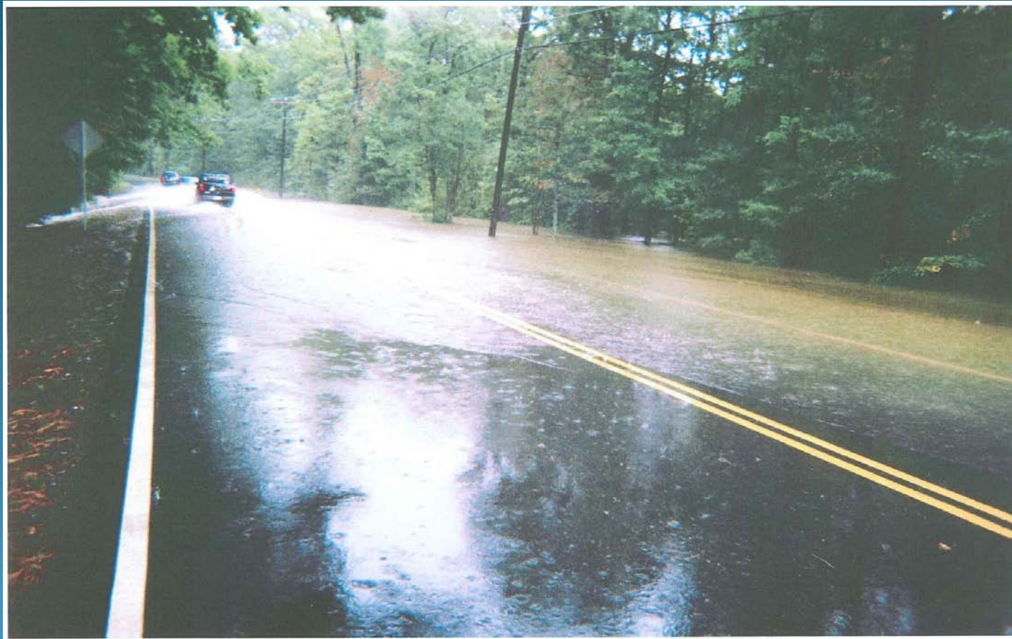
Route 5 under water
