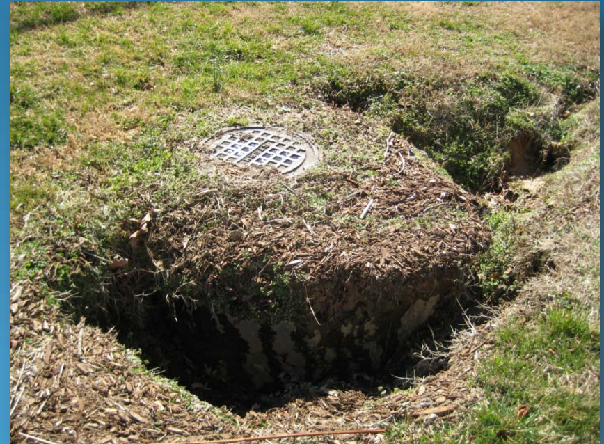
Former sink holes at the JCC-WBG Community Center
