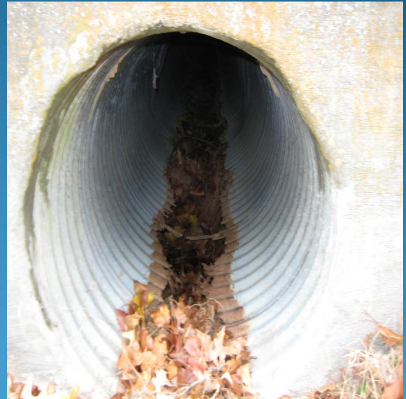
Corroded corrugated metal pipe – Powhatan Shores
