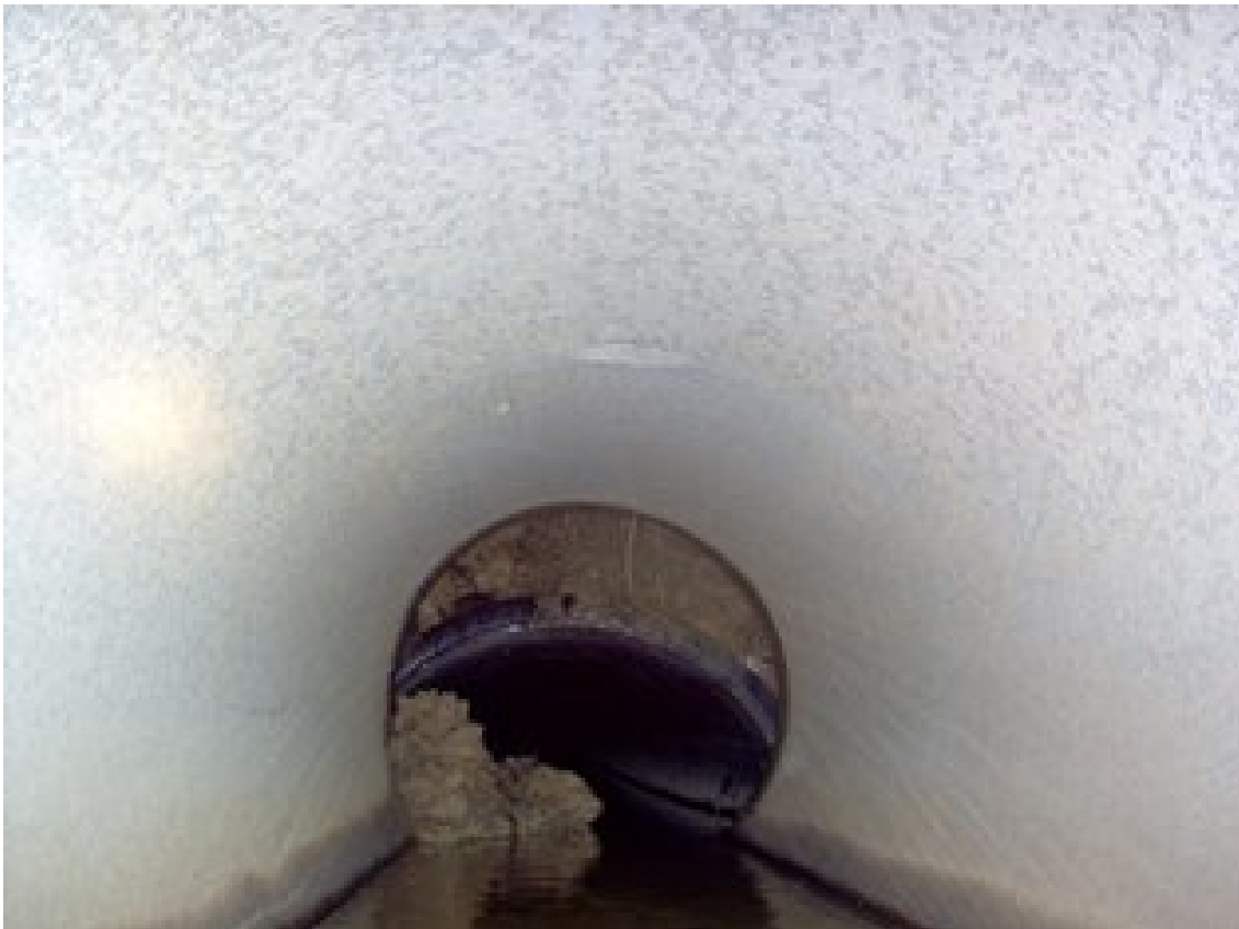
Camera View at location of large sinkhole on General Gookin Court. HDPE pipe at the end of the concrete section in the foreground has separated, deformed and displaced.
