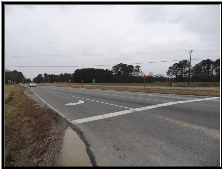
Plate 21. View of project right-of-way at tie-in to Croaker Road, looking west.
