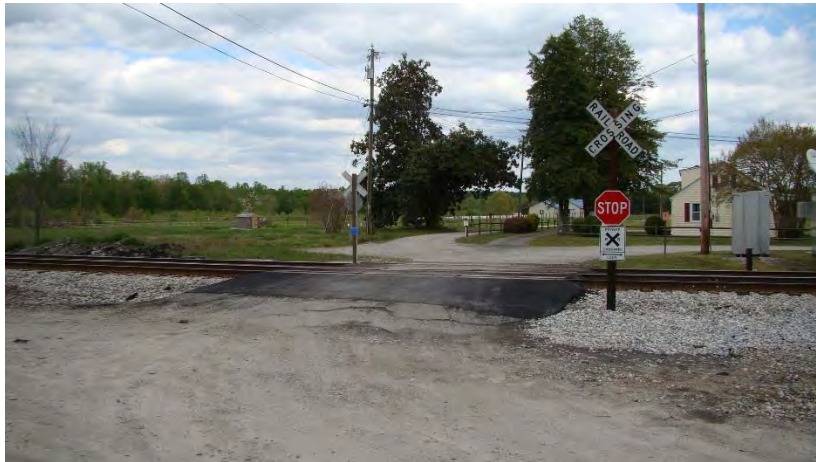
Peach Street railroad crossing
