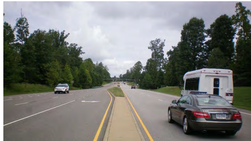
Mooretown Road southeast of Humelsine Parkway
