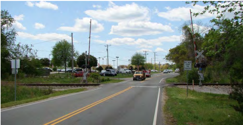
Railroad crossing on Lightfoot Road
