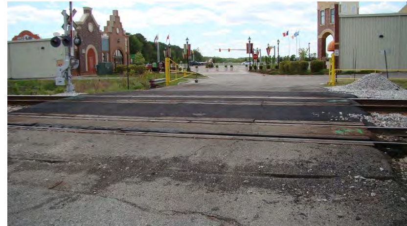
Williamsburg Pottery railroad crossing
