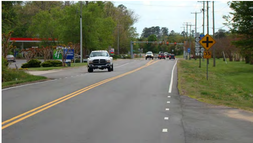
Lightfoot Road looking southeast to Mooretown Road
