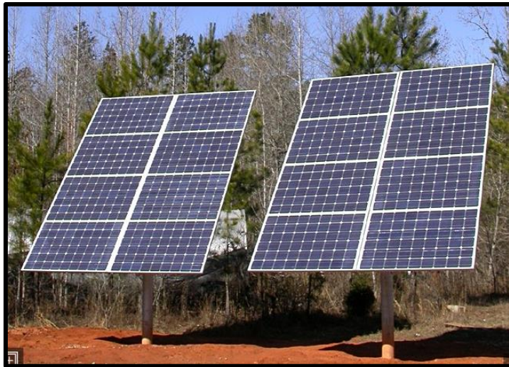
Typical ground-mounted arrays of solar panels
