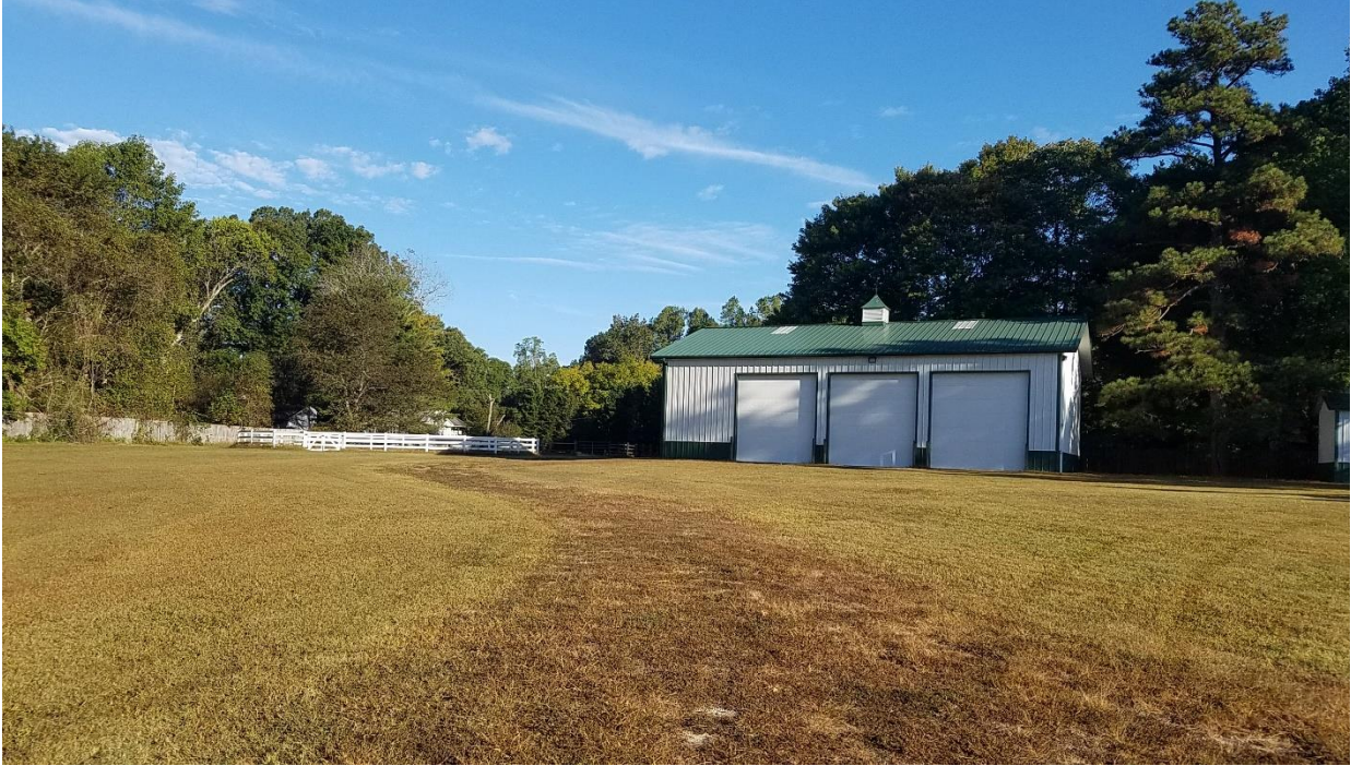
Figure 5. Photo of existing building on site taken while facing north toward Richmond Road. The circular pen is visible to the left.
