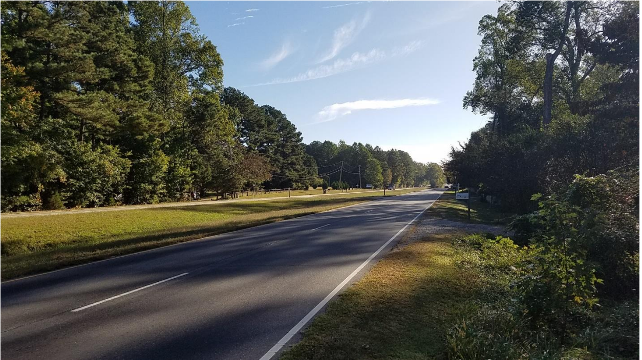
Figure 2: Existing condition along Richmond Road
