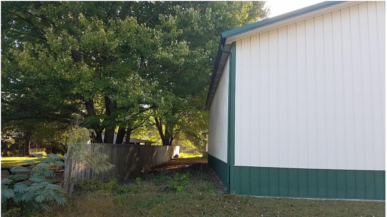
Figure 1: Existing storage building adjacent to 8847 Richmond Road. This building will be re-purposed for Church Office use. Enhanced Landscape Area Type 2 will buffer this building from the residential property
