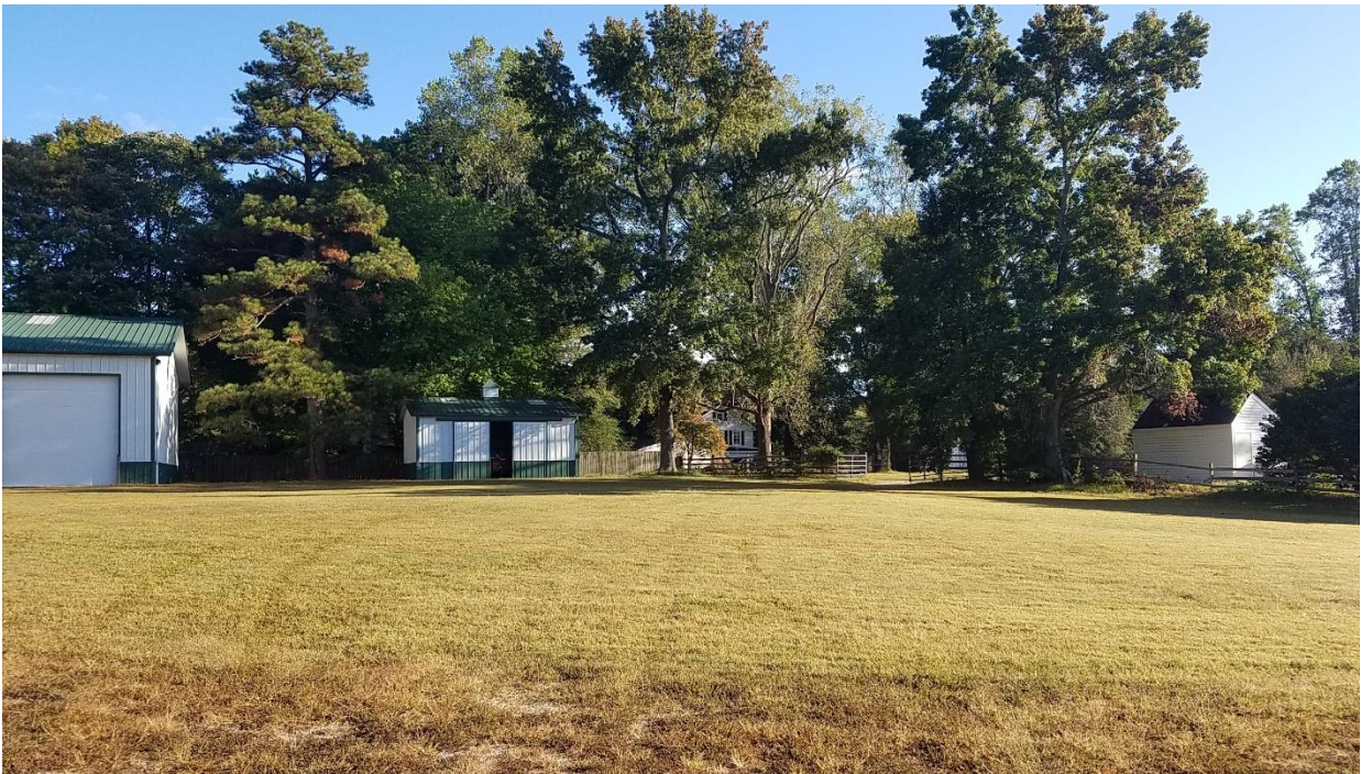
Figure 6. Photo of existing buildings on site taken while facing north towards Richmond Road.
