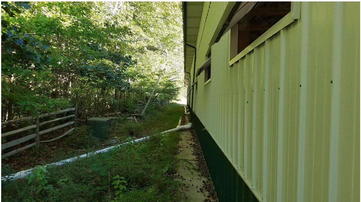
Figure 5: Existing condition between existing indoor riding ring and adjacent property. This building will be converted to the main church building. Enhanced Landscape Area Type 2 will be applied here.
