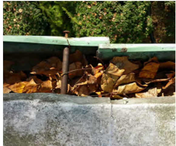
Gutters at porch roof needing repair
