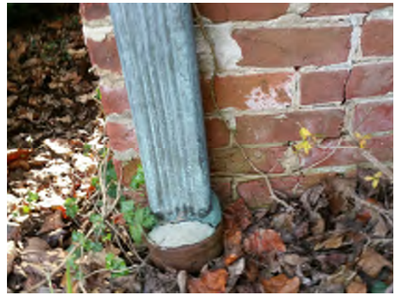
Downspout into underground storm pipe
