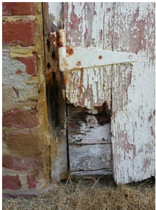
Smokehouse door deterioration
