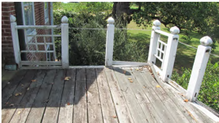
Deteriorated second floor deck and railing
