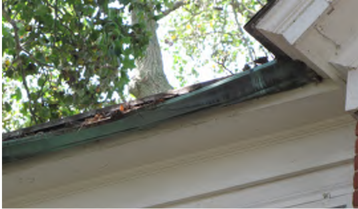
Damaged gutter at porch
