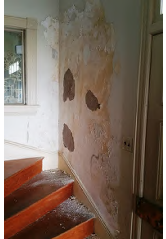
Plaster damage from moisture issues
