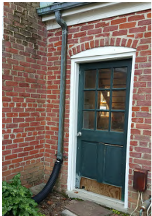
Deteriorated garage door
