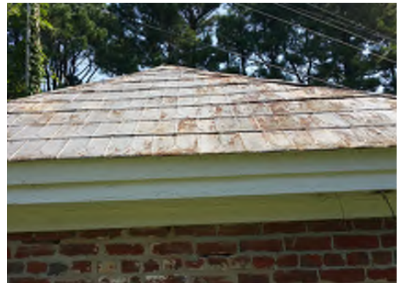
Smokehouse roof deterioration
