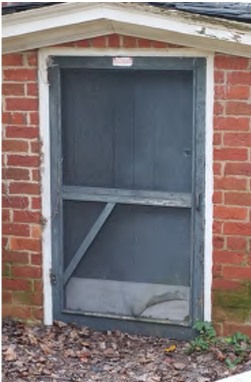
Screen Door deterioration at bulkhead
