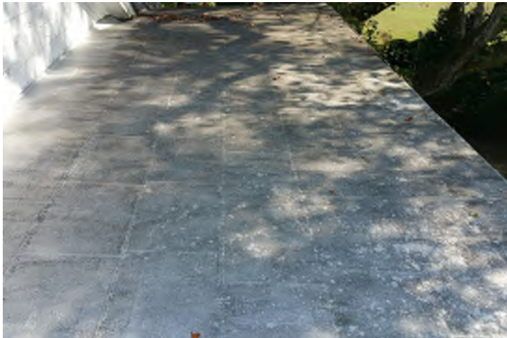
Flat seam metal roof at porch
