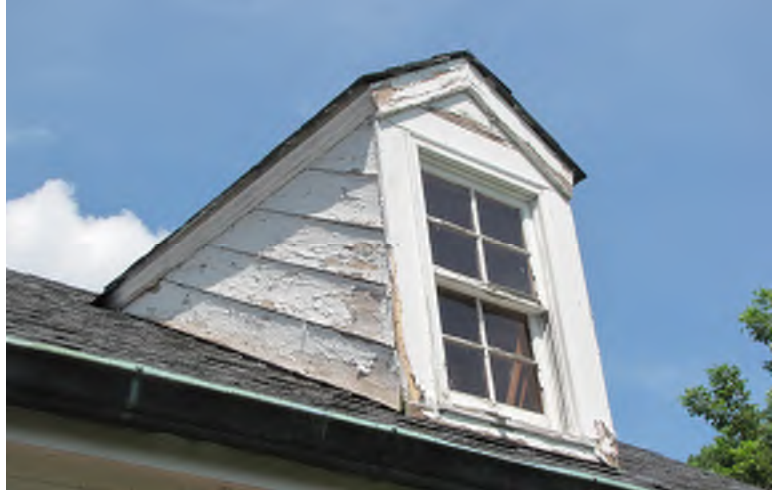
Wood damage at garage dormer
