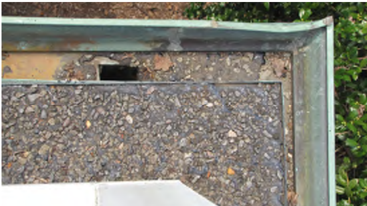
Built-up roof under second floor deck
