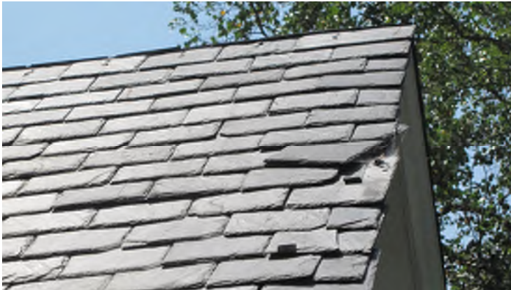
Damaged slate
