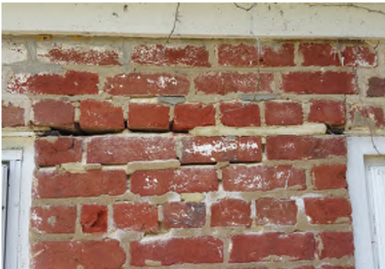
Servant Quarters improper mortar repairs & corroded lintel
