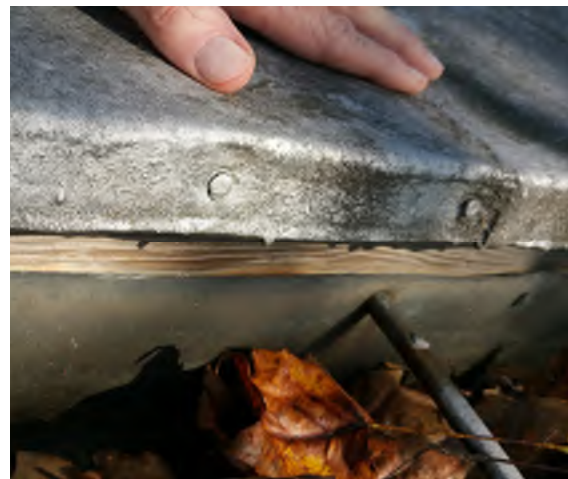
Rework detail at porch roof edge/gutter
