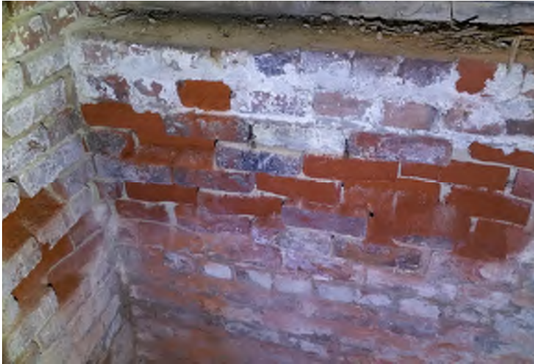
"Rising Damp" deterioration in basement
