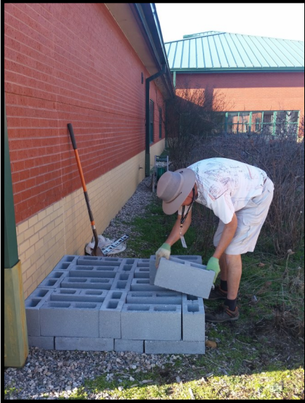
Step 1: Build a sturdy base to hold the water tank. This tank is 500 gallons. That's more than 4,200 lbs. of water!
