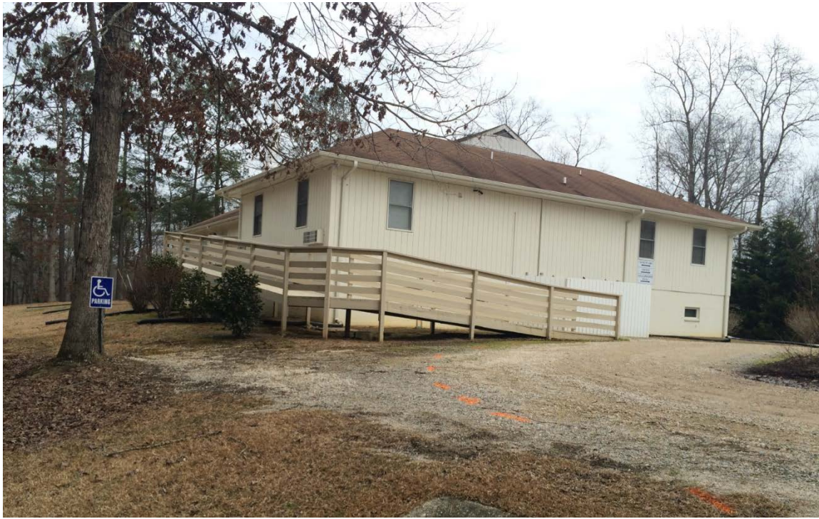
Figure 1. Photo of existing church as viewed from upper gravel parking area.
