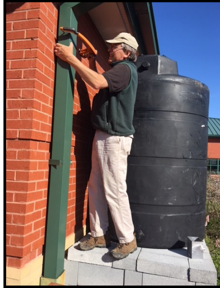
Step 2: Cut the downspout and install a diverter to redirect rainwater from the gutters to the tank. When the tank is full the water flows back down the downspout.
