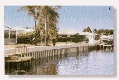
1. This C-LOC vinyl sheet piling wall in Harbor View, Florida, protects the shoreline of a saltwater canal from erosion. Backed by a 50-year limited warranty, the wall is topped with concrete caps which provide additional strength and reduce the costs of installation since fewer tie-back rods are required.
