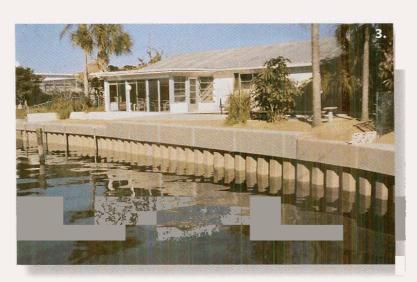
3. A C-LOC vinyl sheet piling wall topped with highly durable concrete caps protects this Florida home's shoreline from erosion and gives the property a neat, finished appearance.
