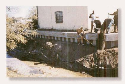
5. The City of Safety Harbor, Florida asked Crane Products Ltd. for help with a creek that was eroding one of its banks next to an office building. Gibson Marine Construction installed a C-LOC vinyl sheet piling wall close to the building and topped it with long-lasting concrete caps that gave it an aesthetically pleasing appearance. The C-LOC panels protected the creek bank from further damage and prevented the building's collapse.
