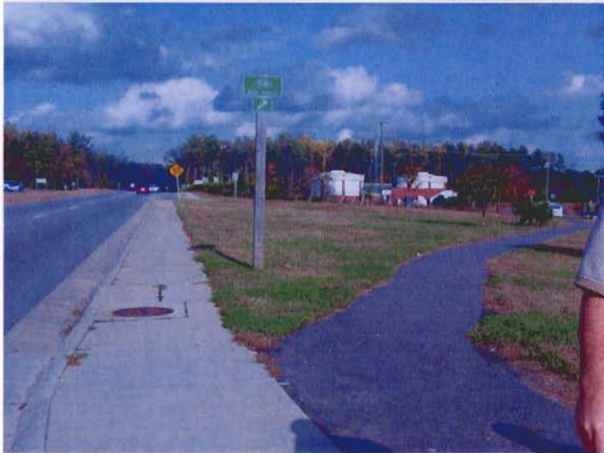
Eastbound bikepath and sidewalk along Monticello Avenue just east of Rt. 199. (Note the need for bikeway pavement marking.)
