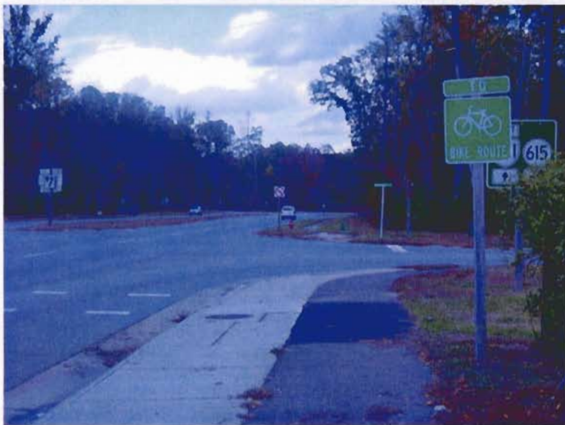
Eastbound bikepath along Monticello Avenue at the intersection of Ironbound Road. Cyclists can turn left and cross Monticello between the white lines or turn right and continue on Ironbound Road. (Note need for directional arrows on the sign and bikeway pavement marking.)
