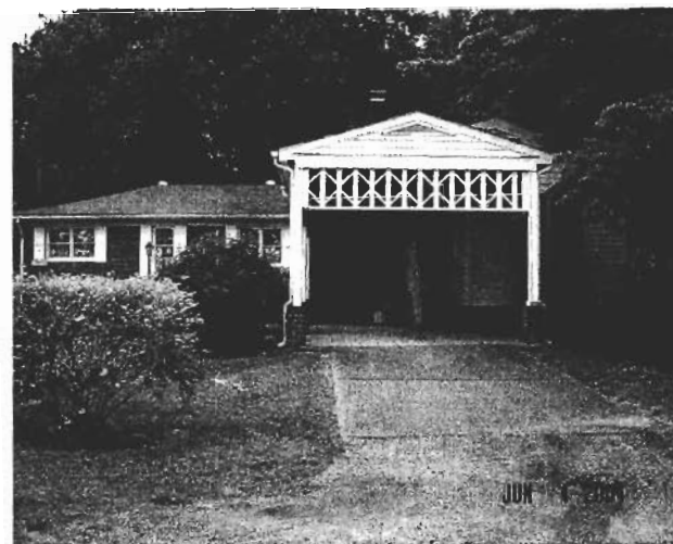
Right: Driveway for the private residence to which the Playhouse is attached.
