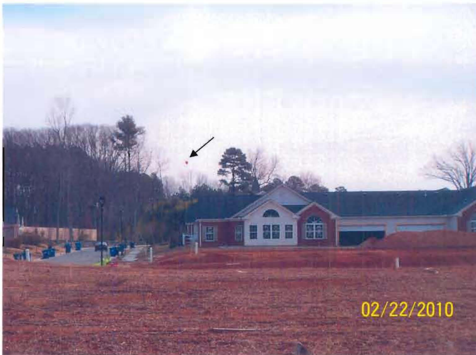
Figure 12: Rear of Villages at Five Forks
