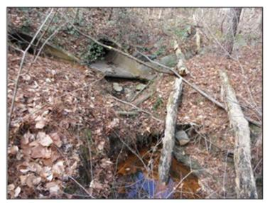
Photo 5: Eroded outfall located at the head of BMP-A1 from Interstate 64 and Croaker Road Interchange
