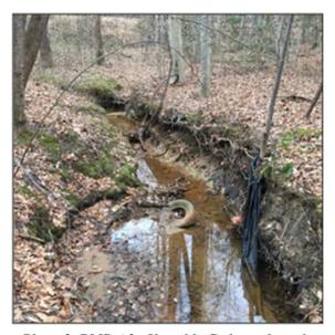
Photo 3: BMP-A2 - Unstable G channel north of Interstate 64 ramp to Croaker Road.
