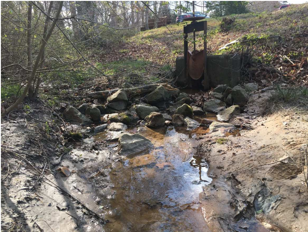
Upper Reach Channel Blockage with Riprap and Excessive Sedimentation
