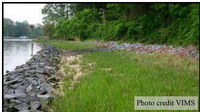
Above: Similar to the photo above, the living shoreline installed along the James River using VACS funds will include rock sills, sand fill, and marsh grass plantings.
