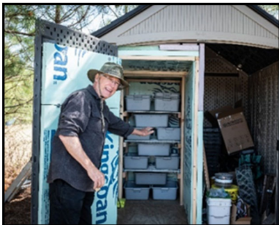
Top Left: Charlie Morse, WCG Executive Director, shows off the repurposed storage shed which was converted to a solar powered walk-in cooler.
