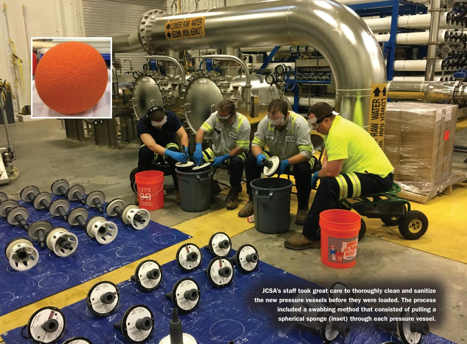
JCSA's staff took great care to thoroughly clean and sanitize the new pressure vessels before they were loaded. The process included a swabbing method that consisted of pulling a spherical sponge (inset) through each pressure vessel.
