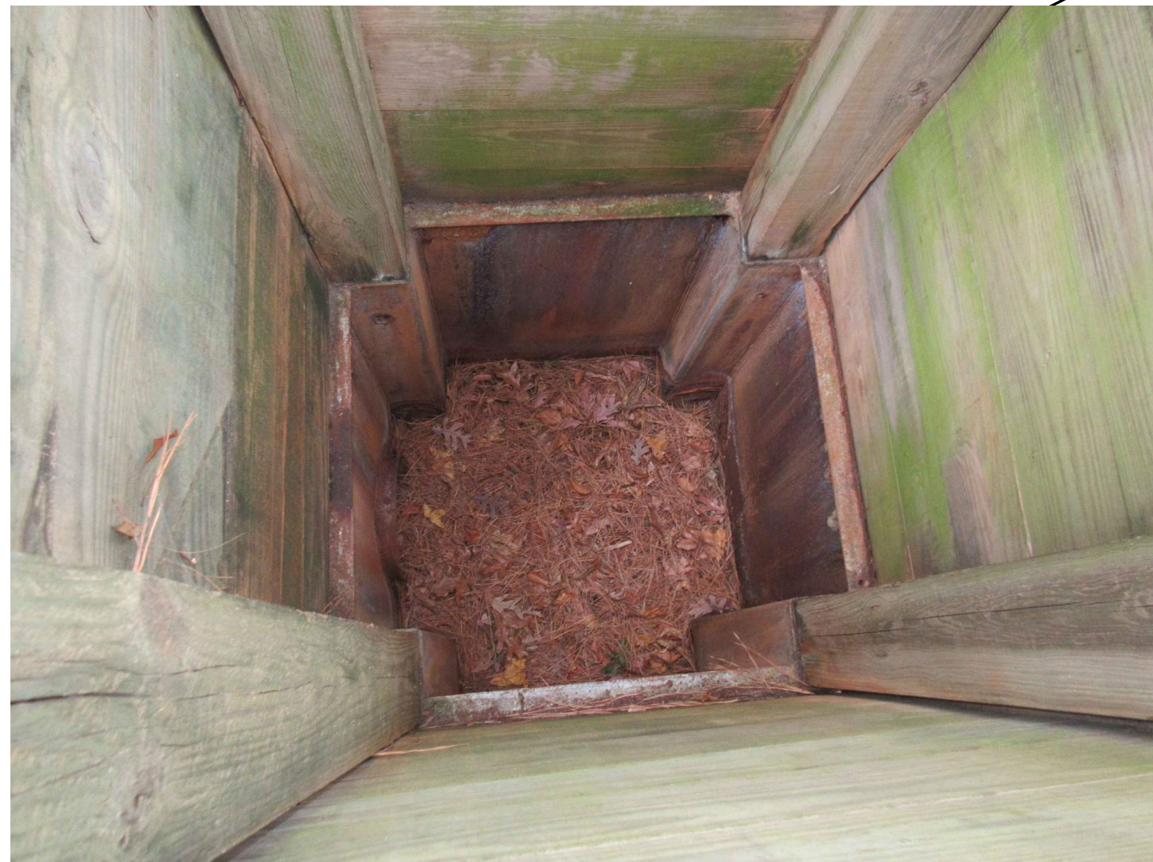
PICTURE 1 - TIMBER WEIR BOX INTERIOR
