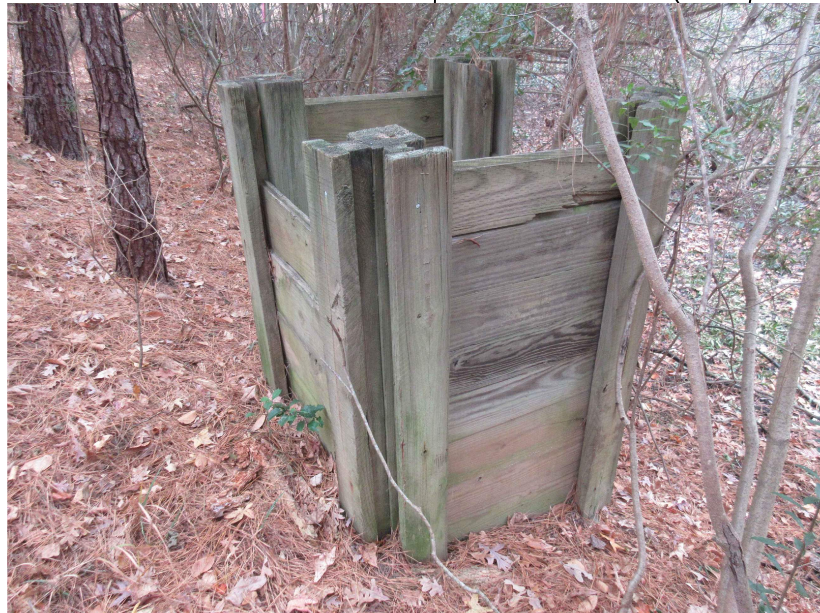
PICTURE 2 - TIMBER WEIR BOX EXTERIOR
