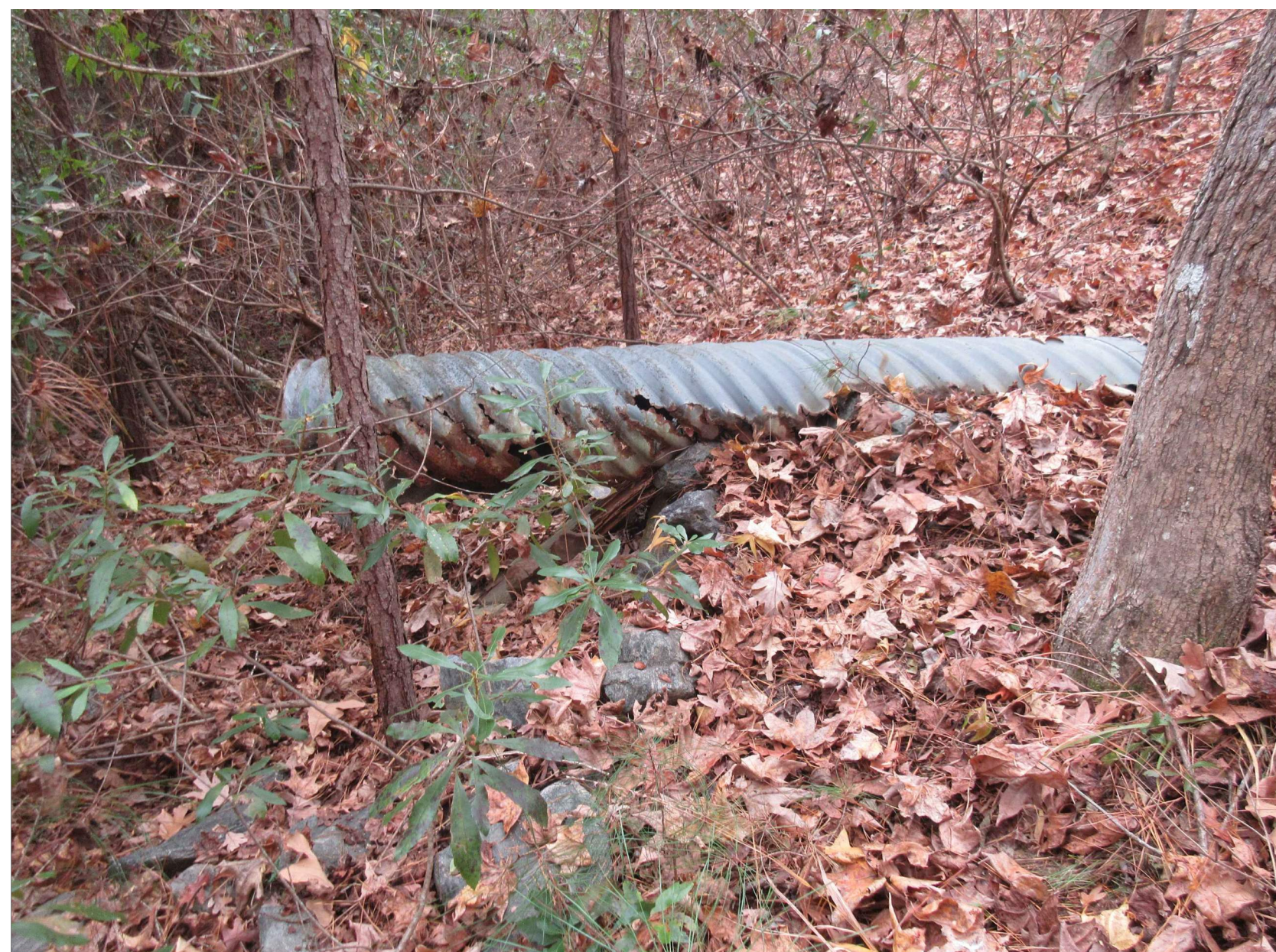
PICTURE 3 - EXISTING PIPE TO BE REPLACED
