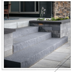
Belgard Highland Stone Wall, Note: Color Of Wall Block & Caps To Match Existing Retaining Wall Materials
