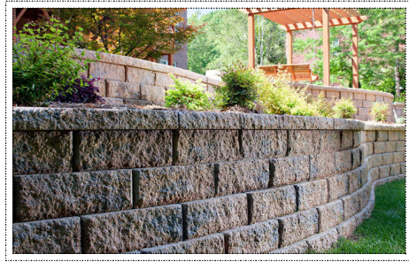
Belgard Highland Stone Wall, Note: Color Of Wall Block & Caps To Match Existing Retaining Wall Materials
