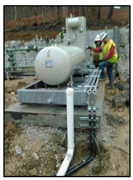
5. Odorant Injection System: Injects odorant in the gas stream to odorize the gas, this allow the detection of a leak by simply smelling. Gas in itself doesn't have an odor.
