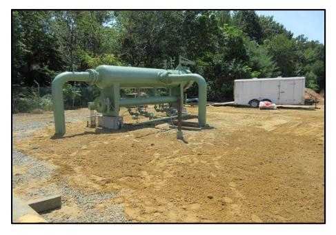
1. Filter Separator: traps any solids/liquids in the system
