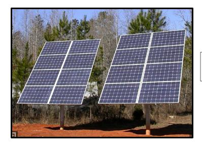
Typical ground-mounted arrays of solar panels
