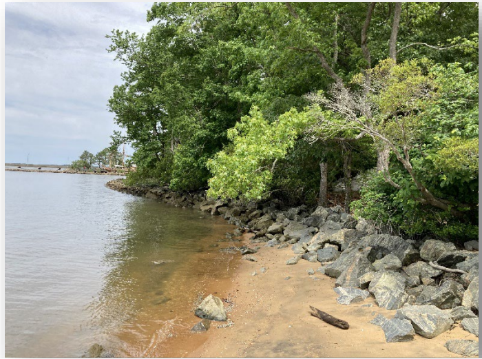
Park staff have already armored shorelines to prevent further damage to resources, but these strategies are only effective in the short term.
