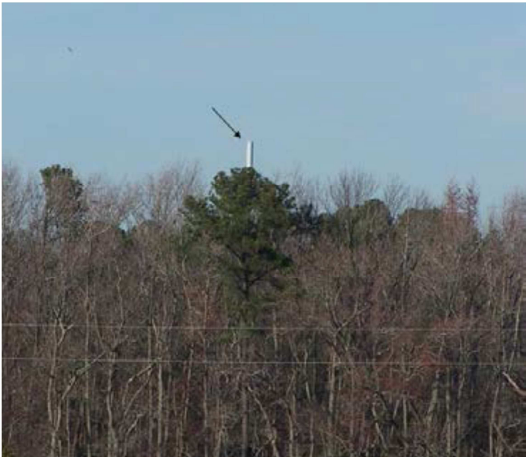
Figure 1: Example of a well buffered slickstick with minimal intrusion
