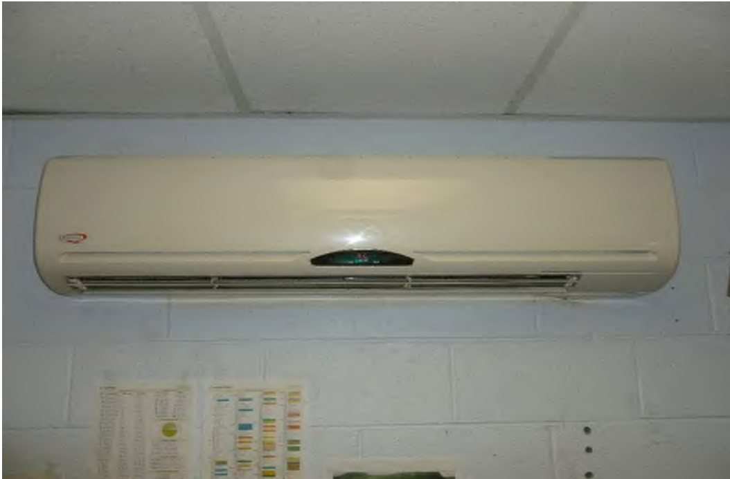
Split System Server Room Air Conditioner Manufacturer: Quietside
