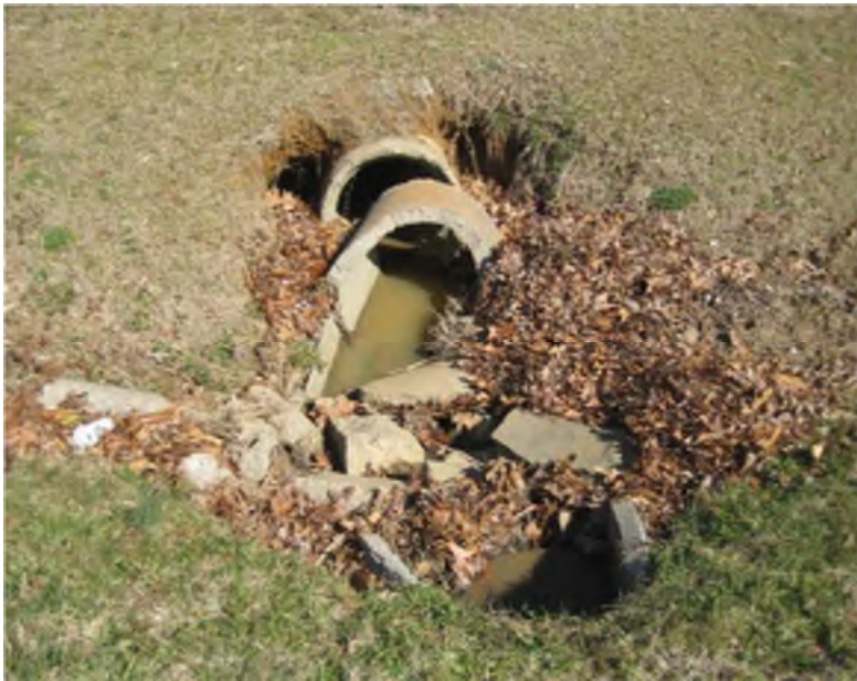
Aging, Failing Storm Drains
