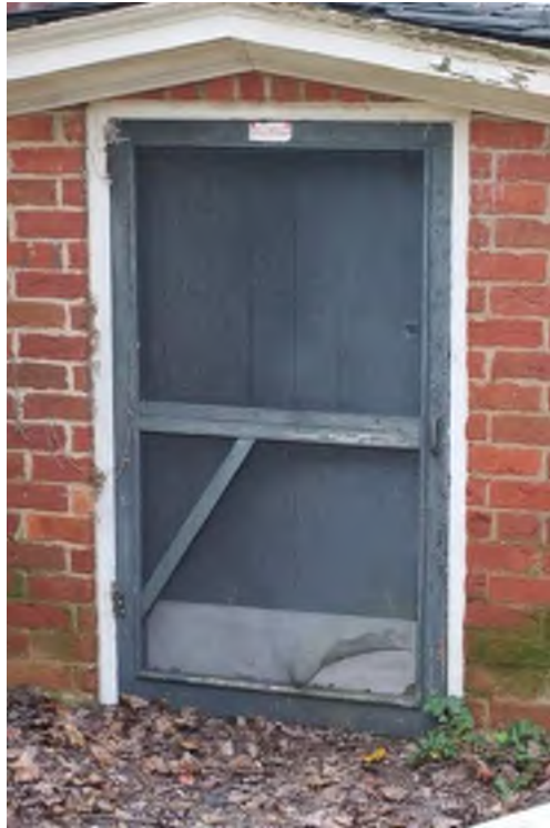
Screen Door deterioration at bulkhead
