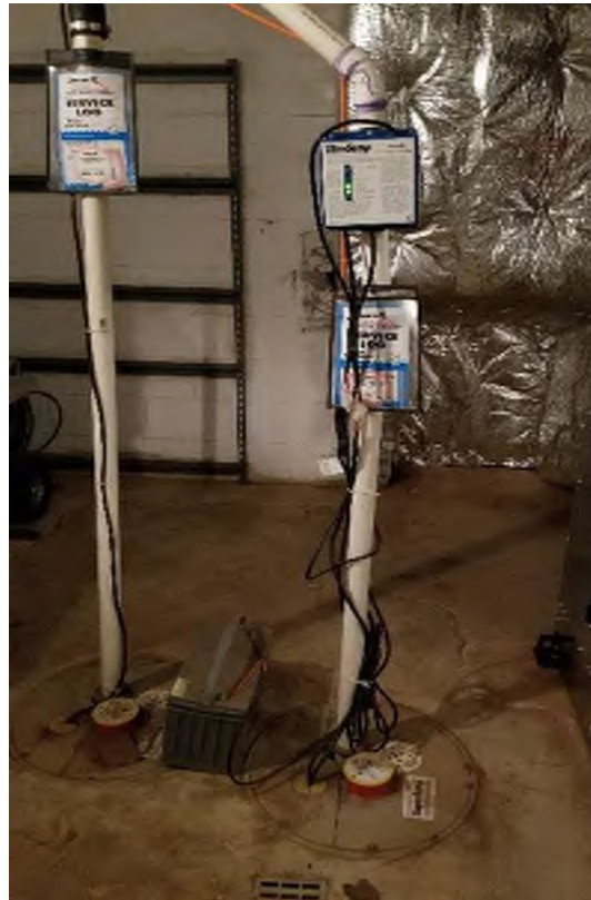
Sump Pump with Battery Backup
