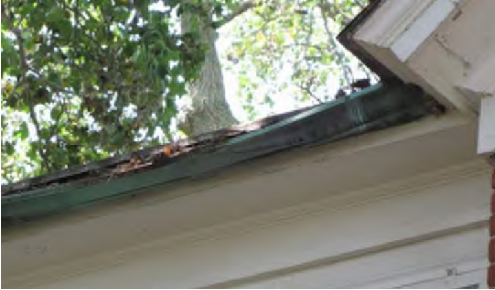
Damaged gutter at porch
