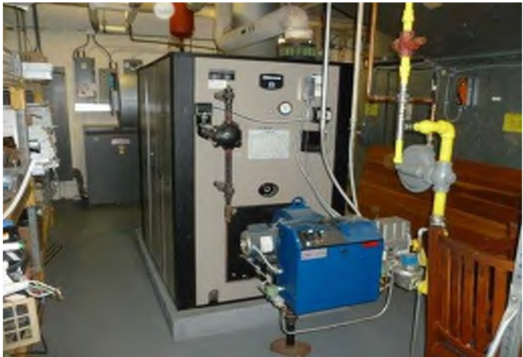
Oil/Natural Gas Fired Boiler (2009) with Conversion to Natural Gas (2013) Manufacturer: Weil-McLain Model No.: 788
