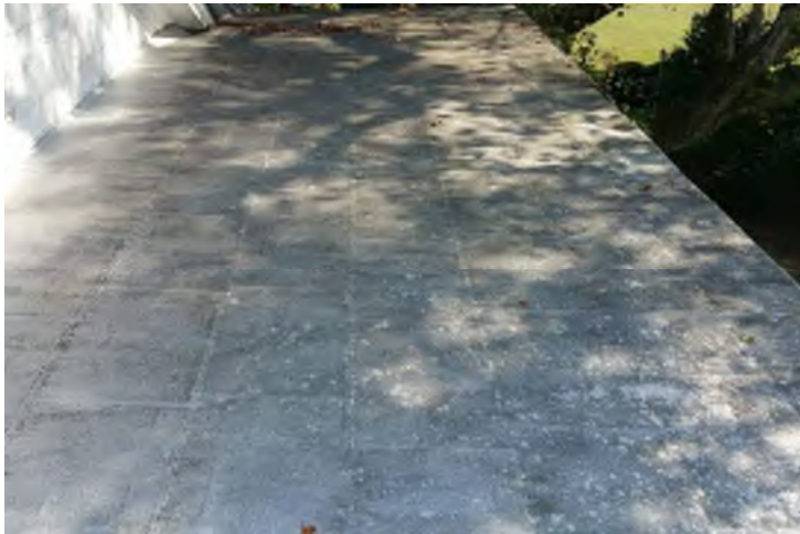
Flat seam metal roof at porch
