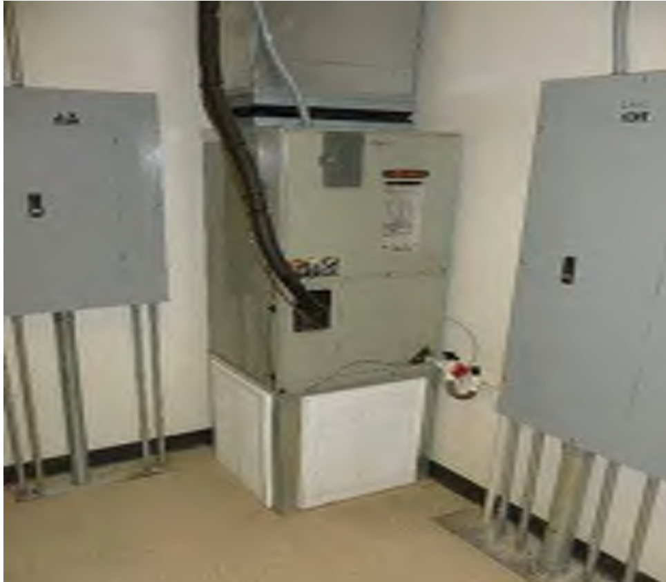
Ducted Split System Heat Pump (Indoor Unit)
