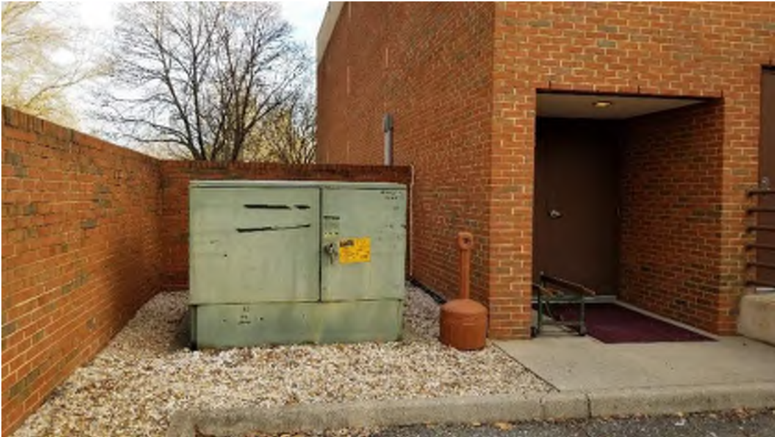
Power Company's Pad Mounted Transformer
