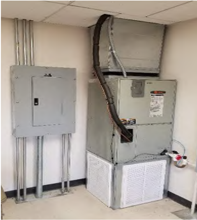
Panelboards in Renovated Area
