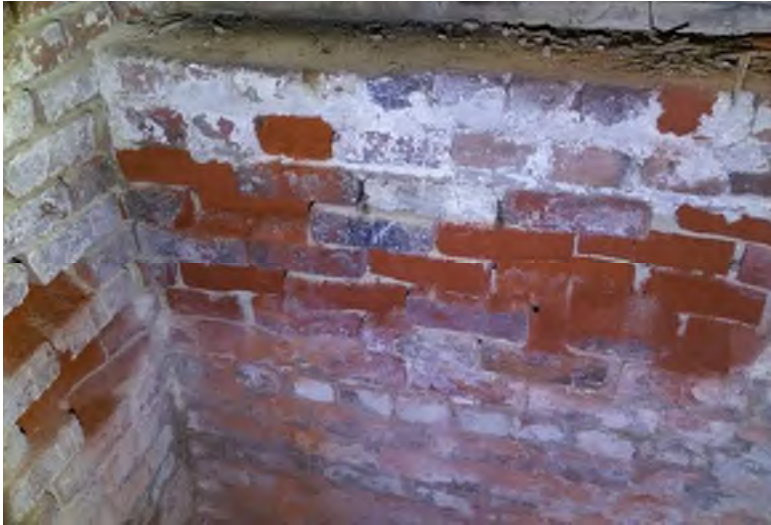
"Rising Damp" deterioration in basement
