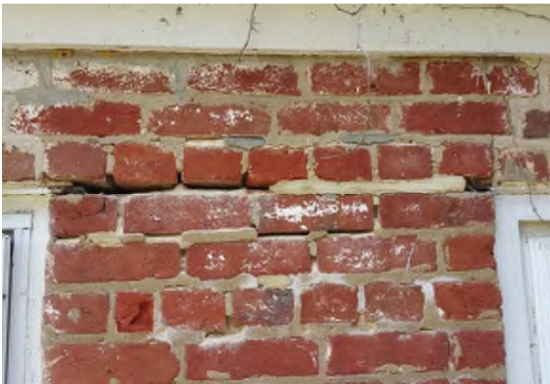
Servant Quarters improper mortar repairs & corroded lintel
