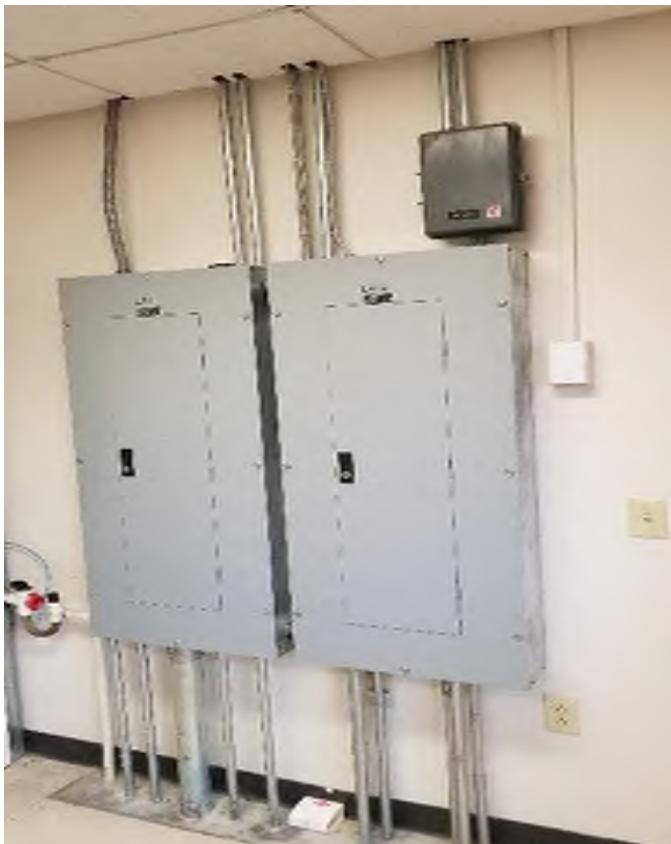
Panelboards in Renovated Area
