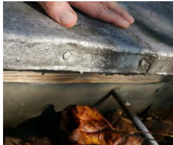
Rework detail at porch roof edge/gutter
