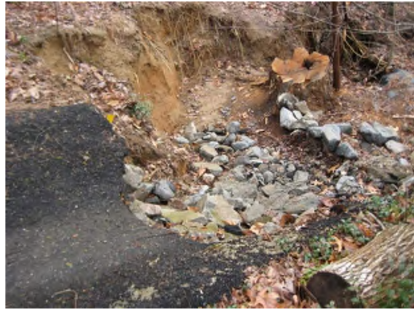
Broken, Eroding Paved Ditches
