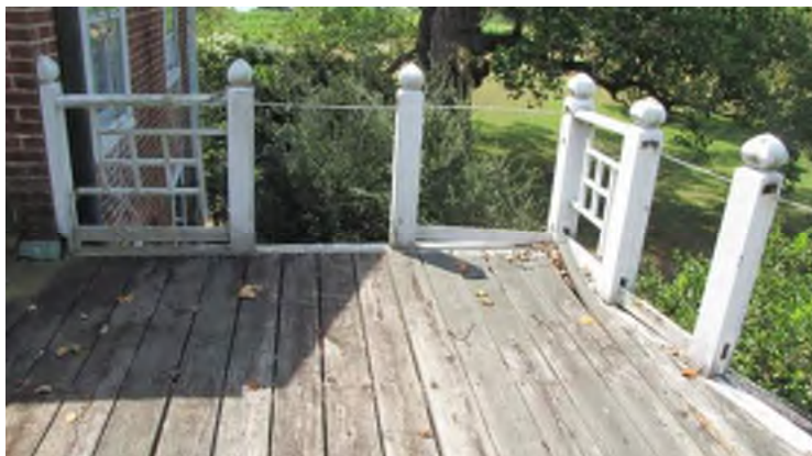
Deteriorated second floor deck and railing
