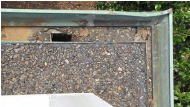
Built-up roof under second floor deck
