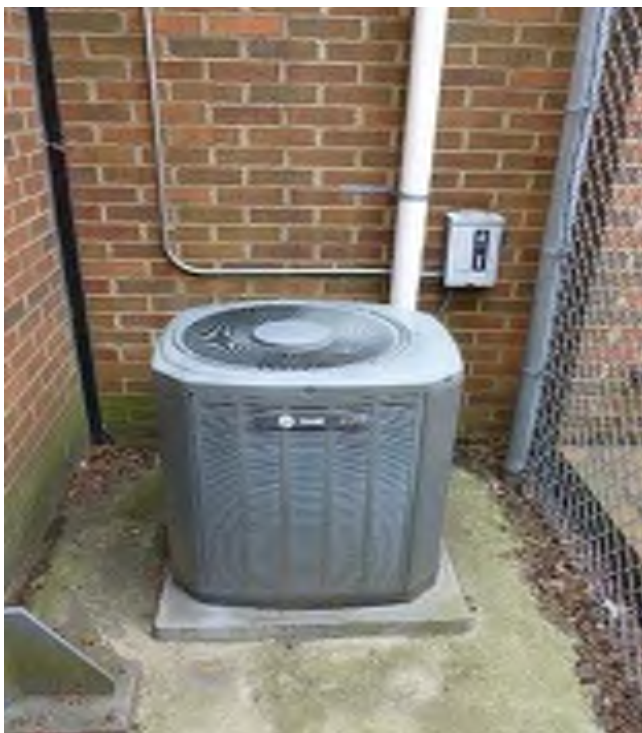
Ducted Split System Heat Pump (Outdoor Unit)
