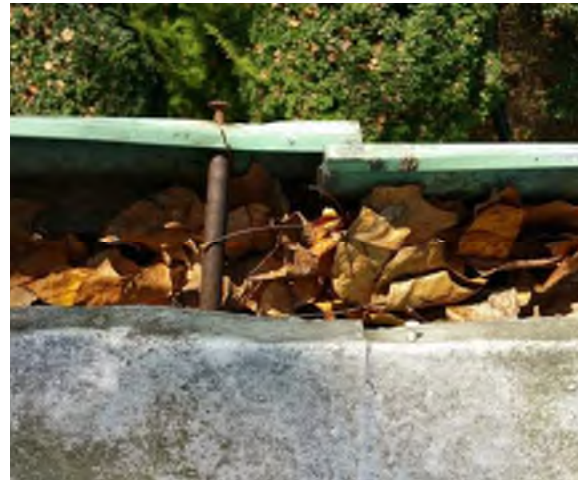
Gutters at porch roof needing repair
