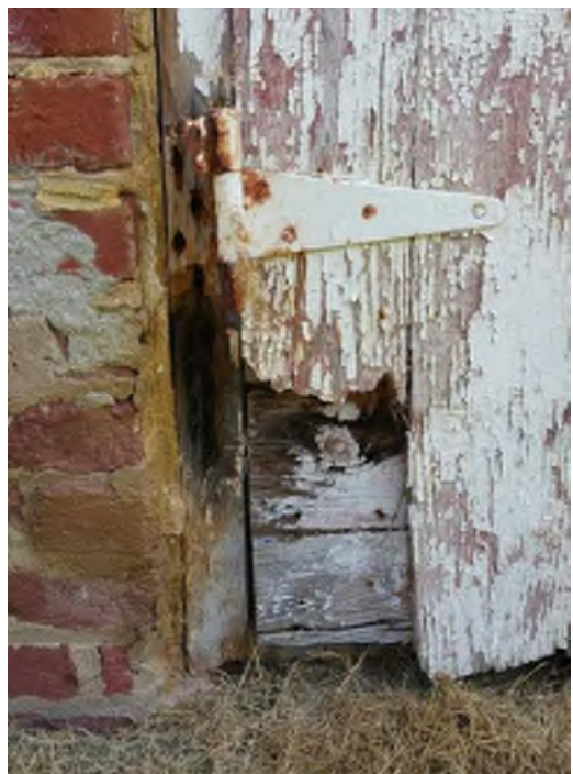
Smokehouse door deterioration
