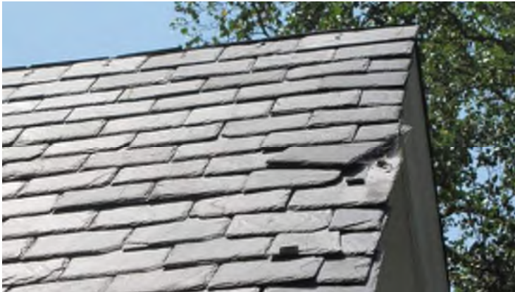
Damaged slate
