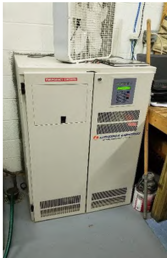
Emergency Battery Backup System (Installed in 2009)
