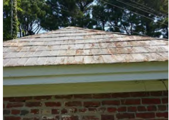
Smokehouse roof deterioration
