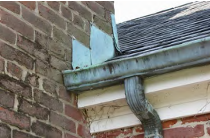
Gutter at garage and main house overflowing
