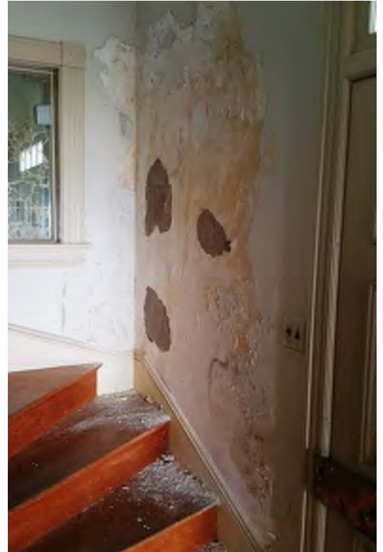
Plaster damage from moisture issues
