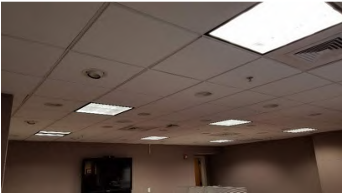
Fluorescent and Incandescent Fixtures in Schell Room
