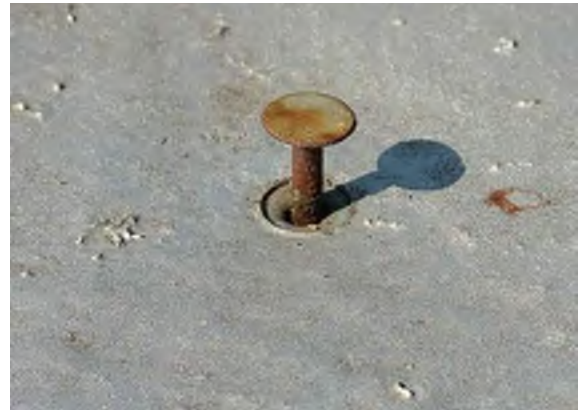
Nail in porch roof repair area
