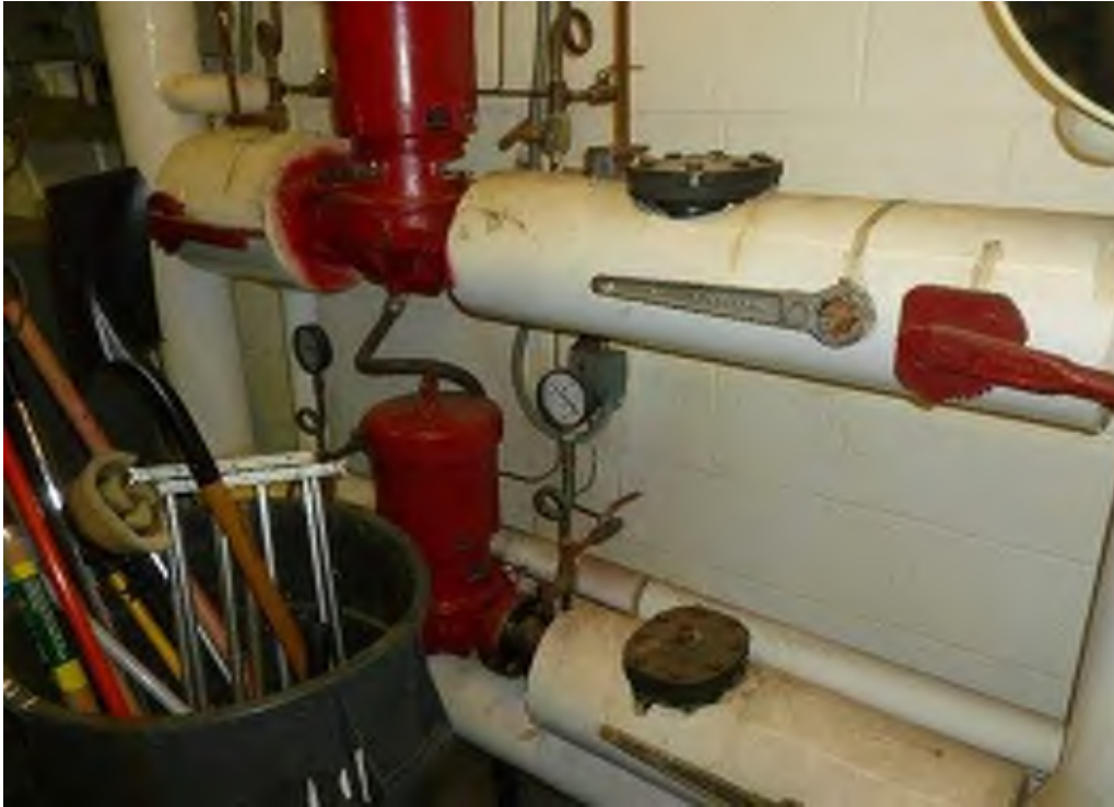
Inline Primary and Secondary Heating Hot Water Pumps Manufacturer: Bell and Gossett
