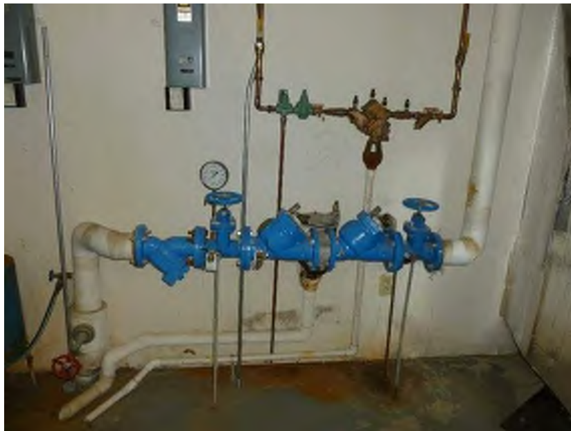
2-1/2" Domestic Water Reduced Pressure Type Backflow Preventer 3/4" Chilled Water Make-Up Reduced Pressure Type Backflow Preventer
