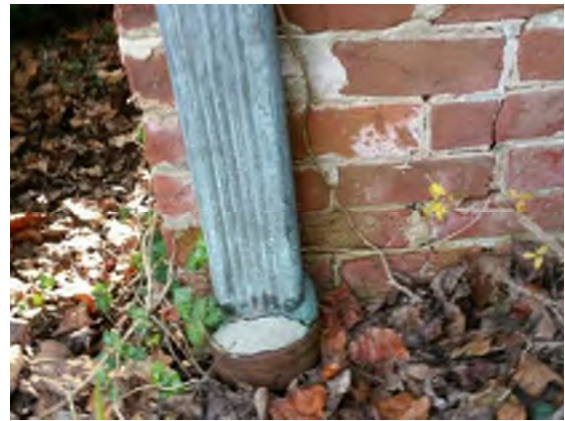
Downspout into underground storm pipe
