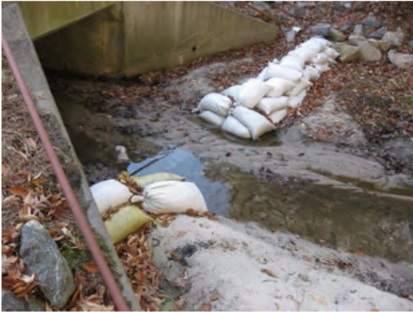
Excessive Erosion from Uncontrolled Runoff
