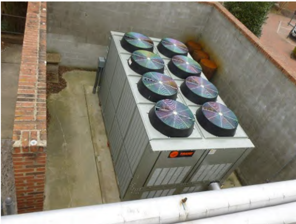
Trane Air Cooled Chiller Manufacturer: Trane (2016) Model No.: CGAM 120F 2NO2 AXD2
