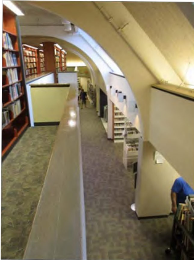
Two Levels of Structural Steel Stacks in 1 ½ Story Space
