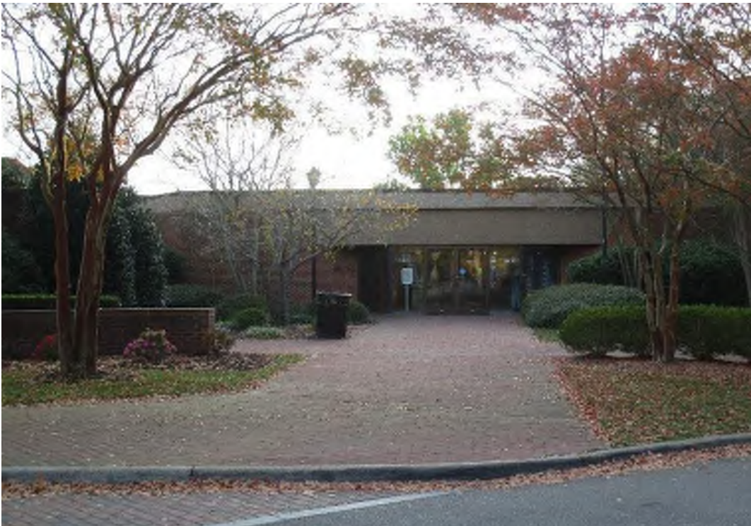
Entry to Auditorium
