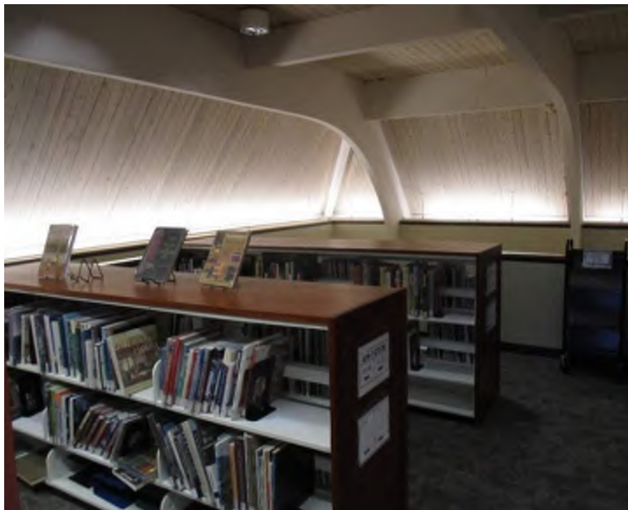
Upper Area of Structural Steel Stacks
