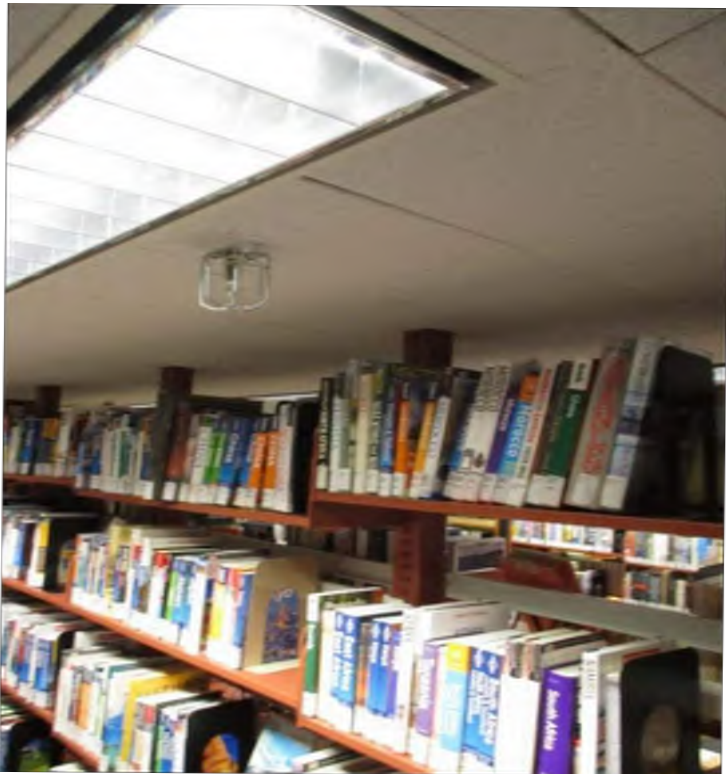
Structural Steel Stacks
