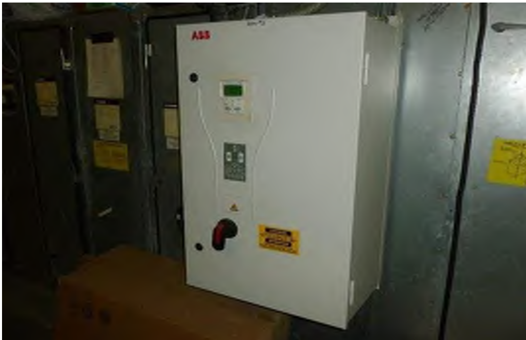
AHU-3 with Variable Frequency Drive Manufacturer: Trane (1997), ABB Supply Fan Frequency Drive (2006)
