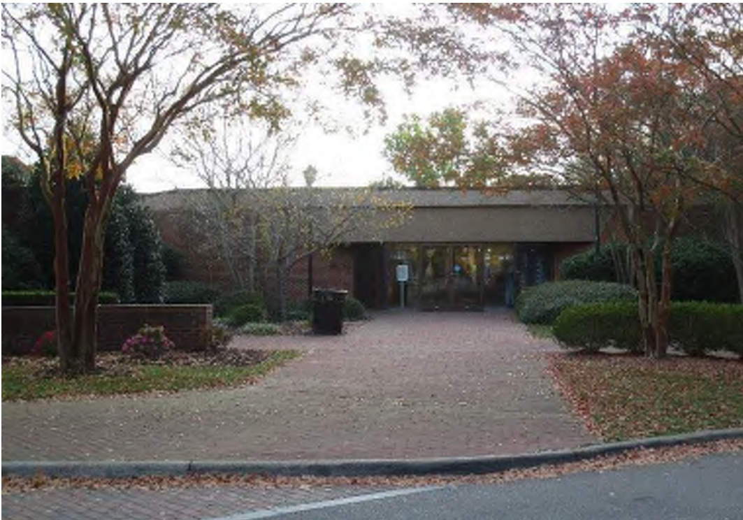
Entry to Auditorium
