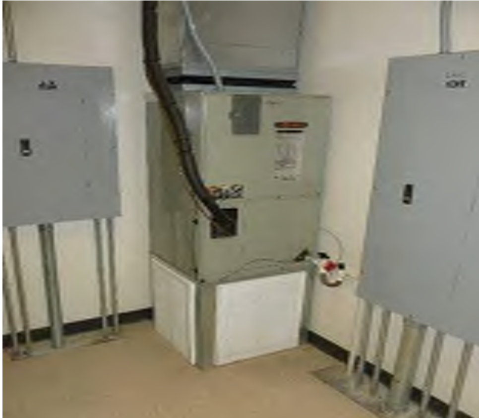
Ducted Split System Heat Pump (Indoor Unit) Manufacturer: Trane (2003) Model No.: TWCO24P130B0
