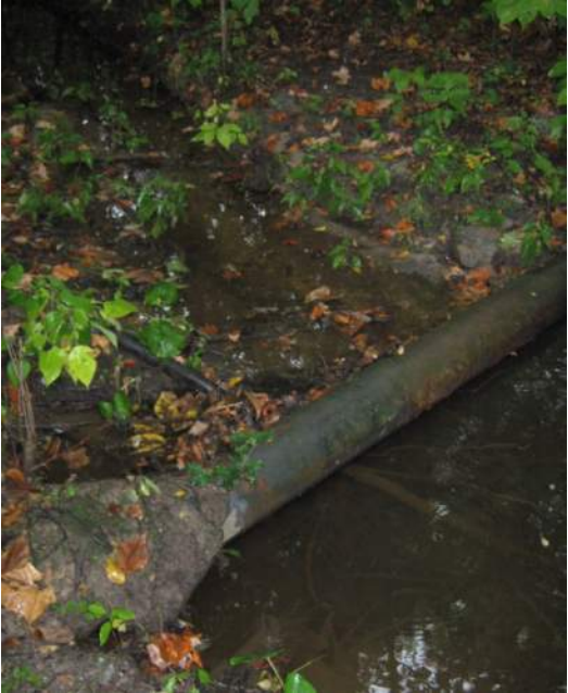
Utility Impacts and Sediment Load, Undercutting and Instability
