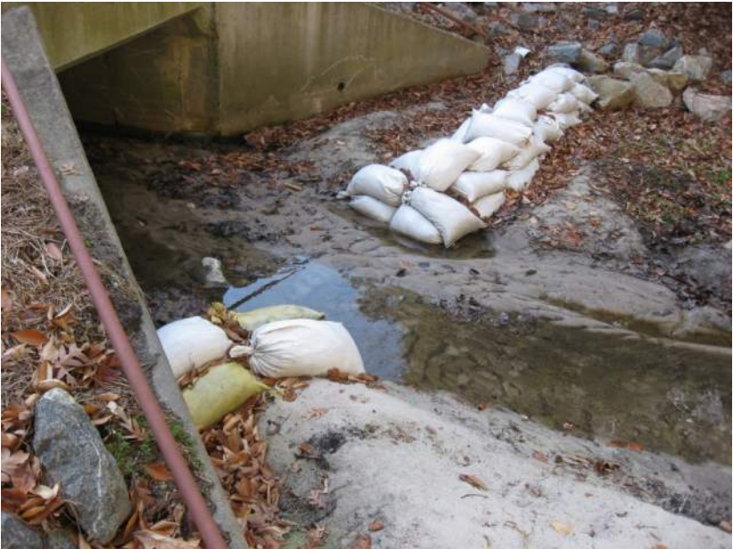
Excessive Erosion from Uncontrolled Runoff
