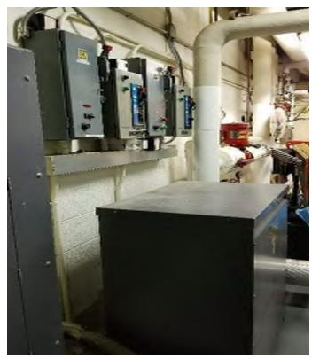
Bank of Disconnect Switches Installed behind Dry Type Transformer (Code Violation
