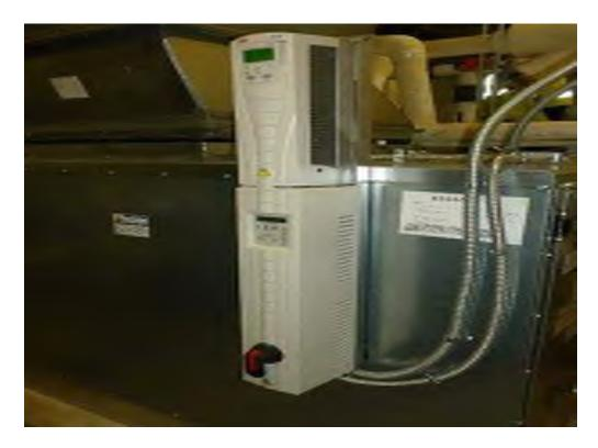
AHU-1 with Variable Frequency Drive
