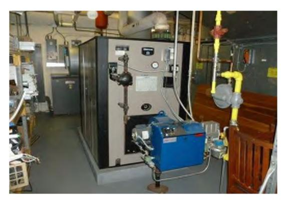
Oil/Natural Gas Fired Boiler (2009) with Conversion to Natural Gas (2013)
