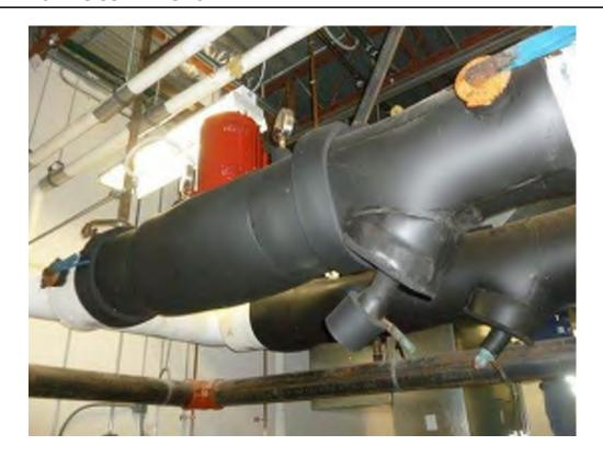
Inline Primary and Secondary Chilled Water Pumps Manufacturer: Bell & Gossett
