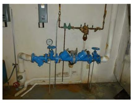
2-1/2" Domestic Water Reduced Pressure Type Backflow Preventer 3/4" Chilled Water Make-Up Reduced Pressure Type Backflow Preventer
