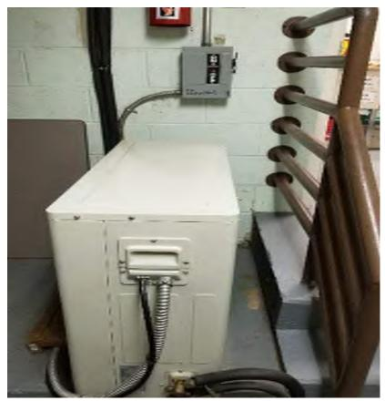
Disconnect Switch for Mini-Split is Installed Behind Unit (Code Violation)
