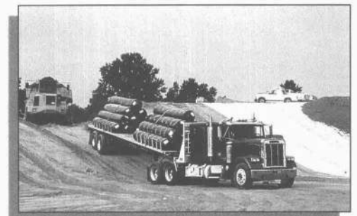
One truckload of GCLs covers the same area as approximately 150 truckloads of compacted clay.
