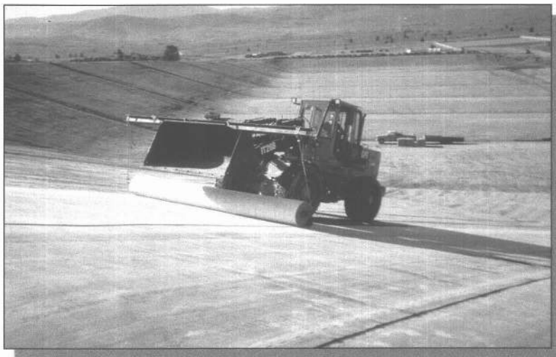
Bentomat installation in a landfill liner system with a 3H:1V slope.
