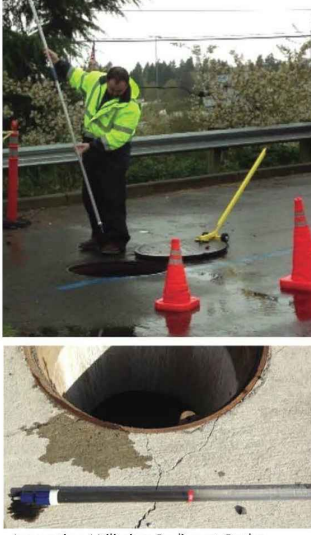
Inspection Utilizing Sediment Probe
