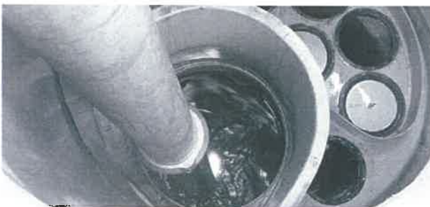
Vacuuming Sump Through MAW
