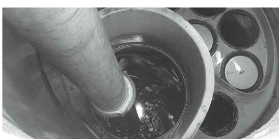
Vacuuming Sump Through MAW
